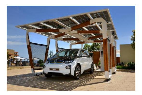
Electricity from the <u>solar panels</u> is directed to a wallbox that not only manages the flow of electricity, i.e. directing it to a hose with a nozzle attachment, but shows usage and allows for routing power to the house when the car's battery is fully charged.
