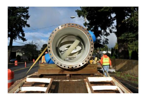
Lucid Energy has developed a renewable energy system that makes use of water moving through pipelines. The company's LucidPipe Power System converts pressure in water pipelines into electricity. They have a patented, lift-based turbine technology and last month they made news in a project involving Lucid Energy, the Portland Water Bureau and Portland General Electric. A 200kW LucidPipe Power System installed
