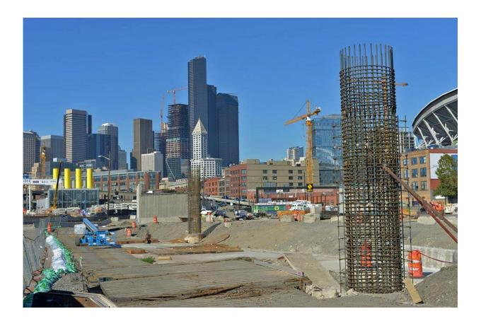
Two super earthquake-resilient columns designed by the University of Nevada, Reno are part of a new exit bridge ramp on a busy downtown Seattle highway. They are built to shake and flex in a large earthquake and remain standing and usable. Credit: Washington Department of Transportation.
