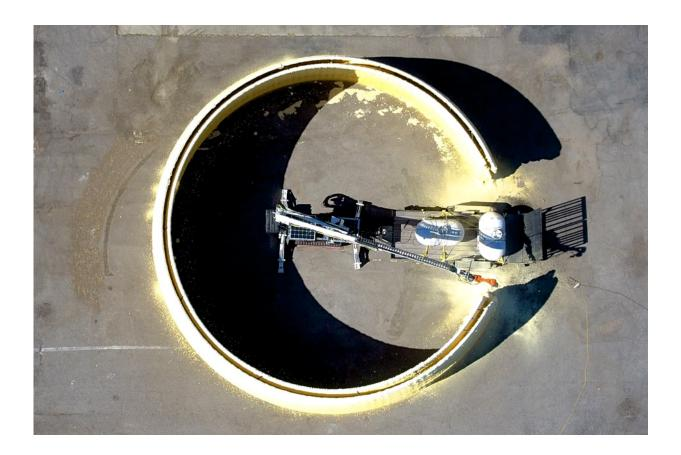
MIT researchers have designed a system that can 3-D print the basic structure of an entire building. The system consists of a tracked vehicle that carries a large industrial robotic arm, which has a smaller, precision-motion robotic arm at its end. Credit: Steven Keating, Julian Leland, Levi Cai, and Neri Oxman/Mediated Matter Group
