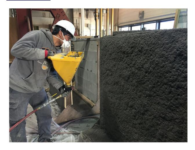
Plastering a wall with seismic-resistant concrete. Credit: UBC
