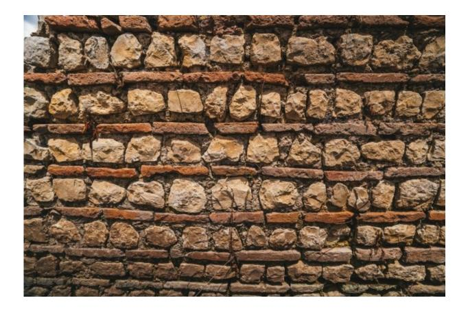
Romans built structures with volcanic ash or recycled materials, like brick fragments, to strengthen the concrete, as seen in this wall in Privernum. This method is more sustainable and has less embodied carbon than modern cement mixtures. Credit: Lillie Paquette
