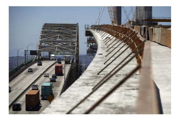
In this July 2, 2018, photo, traffic moves on the old Gerald Desmond Bridge next to its replacement bridge under construction in Long Beach, Calif. The new Gerald Desmond Bridge stretching over the Port of Long Beach is being built with about 75 seismic sensors called accelerometers. They'll measure the forces imparted on the bridge during an earthquake. It's slated to open next year. (AP Photo/Jae C. Hong)
