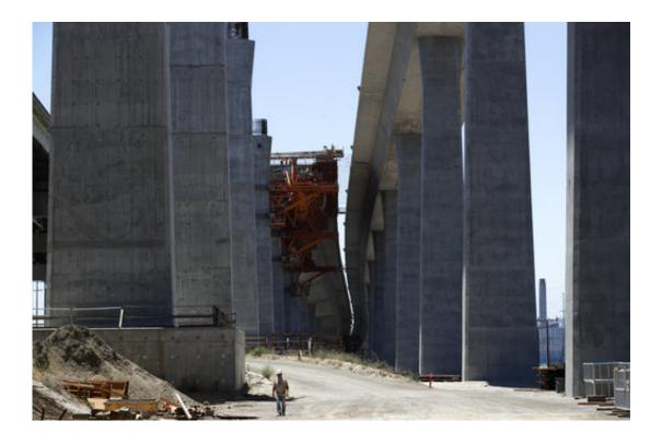
In this July 2, 2018, photo, a worker walks under the new Gerald Desmond Bridge under construction in Long Beach, Calif. The bridge, which will stretch 8,800 feet over the Port of Long Beach when it opens next year, is being built with about 75 seismic sensors that will measure the forces imparted on the span when one of several nearby faults set off an earthquake. (AP Photo/Jae C. Hong)
