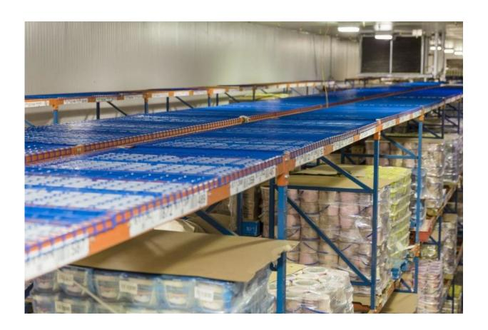
The thermal-energy system being tested in a Bashas' ice cream freezer employs "ice packs" of phase-change materials that can transform repeatedly from liquid to solid and back to liquid again. The materials are encased in plastic and placed on the racks of shelving throughout the storage facility. Credit: Salt River Project
