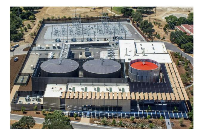
At Stanford's Central Energy Facility, the two larger tanks hold chilled water and the smaller tank holds hot water. Credit: Steve Proehl
