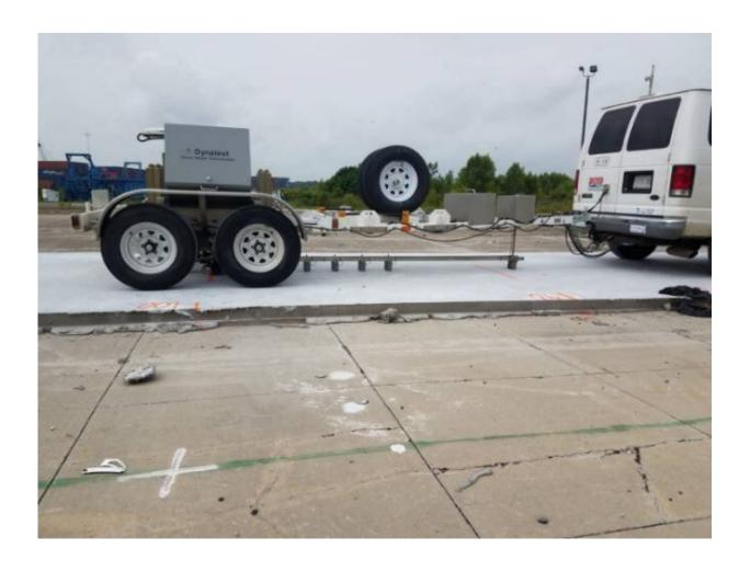
LSU researchers constructed three 60-foot-long overlay sections on top of a section of deteriorated asphalt at the Louisiana Transportation Research Center in order to restore its condition. Credit: LSU College of Engineering
