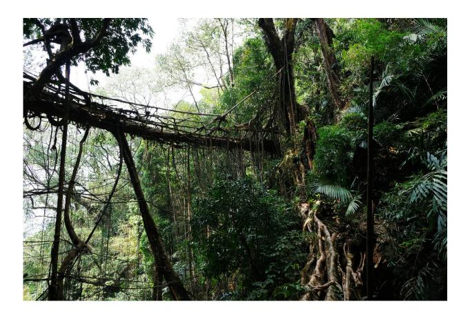
The so-called Meghalaya bridges often lead over steep valleys. Many are secured by railings and handrails also made from the aerial roots. Credit: Ferdinand Ludwig
