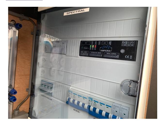
The Fraunhofer ITWM's energy management system goes by the name of Amperix®; myPowerGrid is a platform for microgrids and energy communities. Credit: Fraunhofer ITWM
