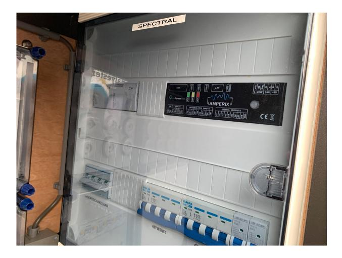
The Fraunhofer ITWM's energy management system goes by the name of Amperix®; myPowerGrid is a platform for microgrids and energy communities. Credit: Fraunhofer ITWM
