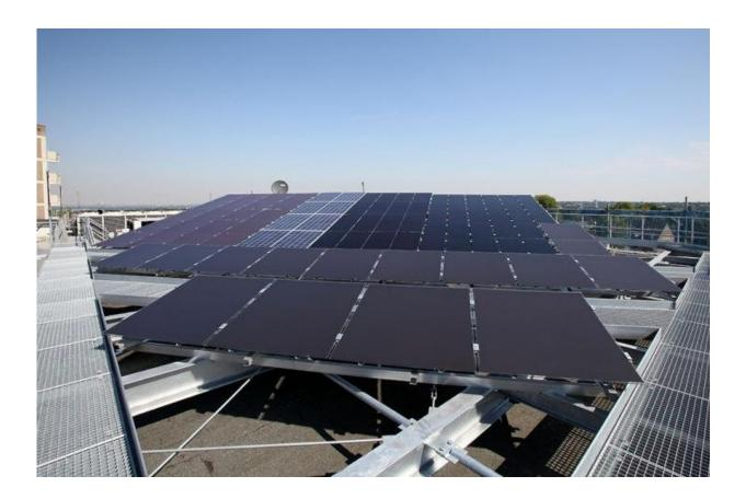
The PV field-testing facility located at the Max Planck Institute for Chemical Energy Conversion (MPI-CEC), located in Mülheim an der Ruhr, Germany. The rooftop installation includes five different inorganic PV technologies. Credit: Thomas Hobirk, MPI-CEC
