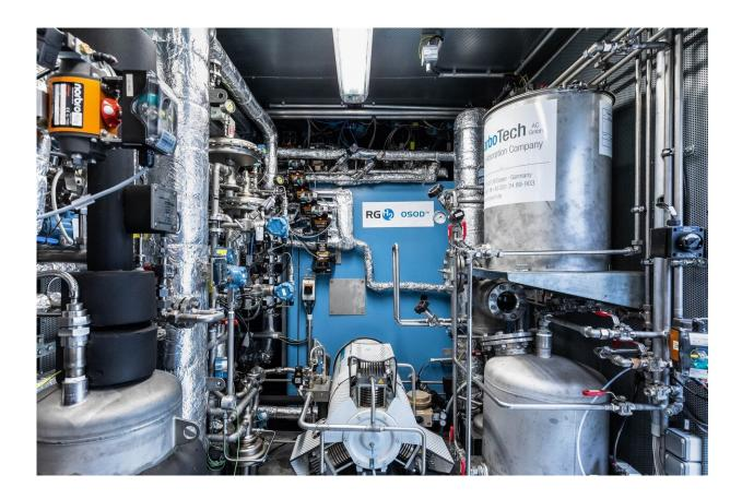
The inner workings of the OSOD H2 generator. The blue cuboid is the core development: a gas furnace with four tubular reactors in which the chemical looping process for hydrogen production takes place. Credit: RGH2
