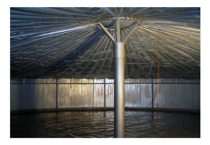
Interior of the test tank. The gas membrane partly lies on the support construction. Credit: Rosemarie Wagner, KIT
