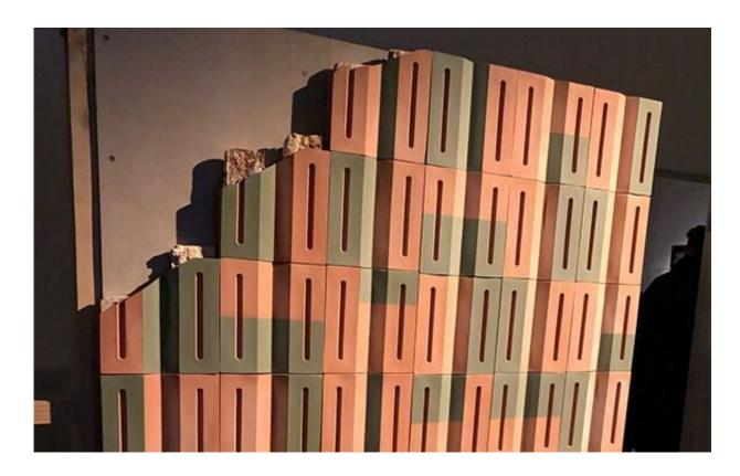
Assembled ceramic tiles with mycelium fill, at Fireless Skin exhibition. Credit: Mehrnoush Latifi
