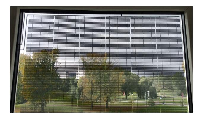
Photovoltaic windows contain embedded solar panels that can harvest electricity while still letting in light. Credit: TNO & NSG Pilkington
