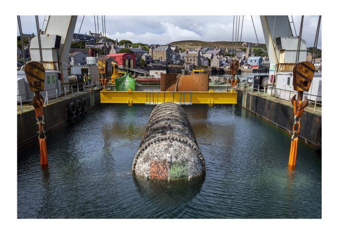
The Northern Isles datacenter was retrieved from the seafloor off Scotland's Orkney Islands and towed partially submerged between the pontoons of a gantry barge to a dock in Stromness, Orkney. A coat of algae, barnacles and sea anemones grew on the datacenter during its two-year deployment. Credit: Jonathan Banks
