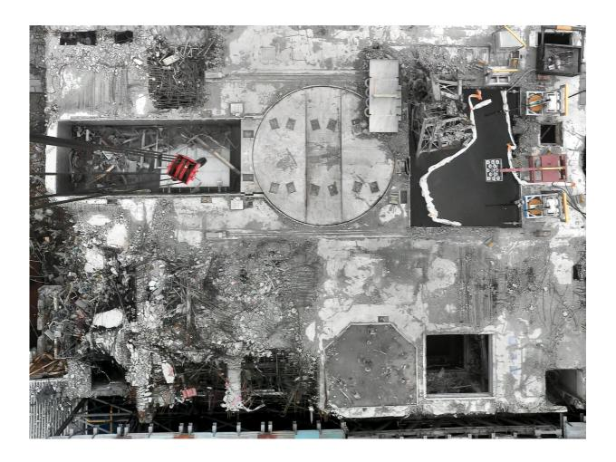
This Jan. 31, 2014, image released by Tokyo Electric Power Company Holdings shows the aerial view of the No. 3 reactor, with its roof blown off and shield plug (circle in the middle) exposed, in Okuma town, Fukushima prefecture, northeastern Japan. A draft investigation report into the 2011 Fukushima nuclear meltdown, adopted by Japanese nuclear regulators Wednesday, Jan. 27, 2021,
