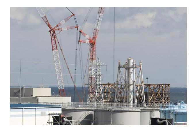
This photo shows the damaged Unit 1 reactor, back, and part of the exhaust stack shared with the Unit 1 and 2 reactors at the Fukushima Daiichi nuclear power plant in Okuma town, Fukushima prefecture, northeastern Japan, Saturday, Feb. 27, 2021. The exhaust stack has gotten its upper half cut off due to safety concerns. (AP Photo/Hiro Komae)
