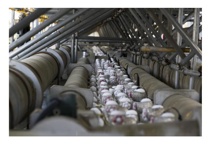
This photo shows a device to freeze dirt to make an underground retention wall to surround nuclear reactors in an attempt to avoid leakage of radioactive water at the Fukushima Daiichi nuclear power plant in Okuma town, Fukushima prefecture, northeastern Japan, Saturday, Feb. 27, 2021. (AP Photo/Hiro Komae)
