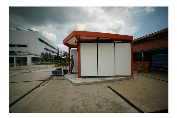
The researchers demonstrated their cooling system by building a pavilion in Singapore featuring a system of chilled tubes enclosed within a condensationpreventing membrane. Credit: Lea Ruefenacht
