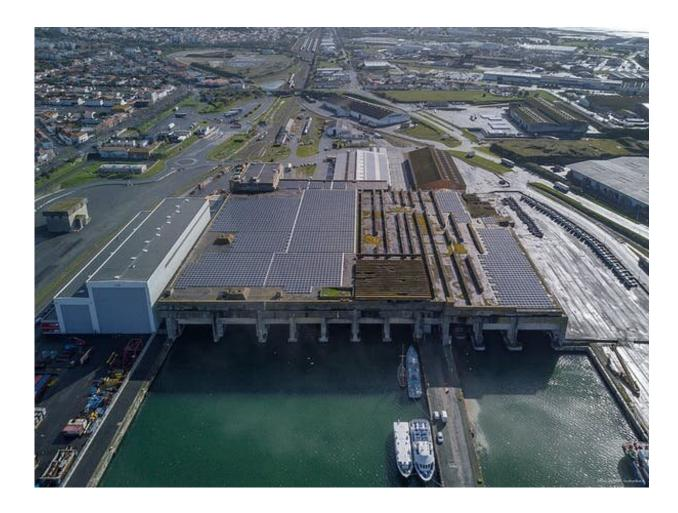
The roof of the submarine base in the La Rochelle port was fitted out with 7,580 solar panels in 2018. Credit: Olivier Benoît, Author provided
