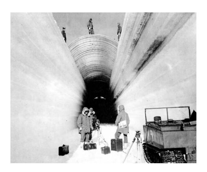
The Camp Century tunnels started as trenches cut into the ice. Credit: <u>U.S. Army</u> <u>Corps of Engineers</u>
