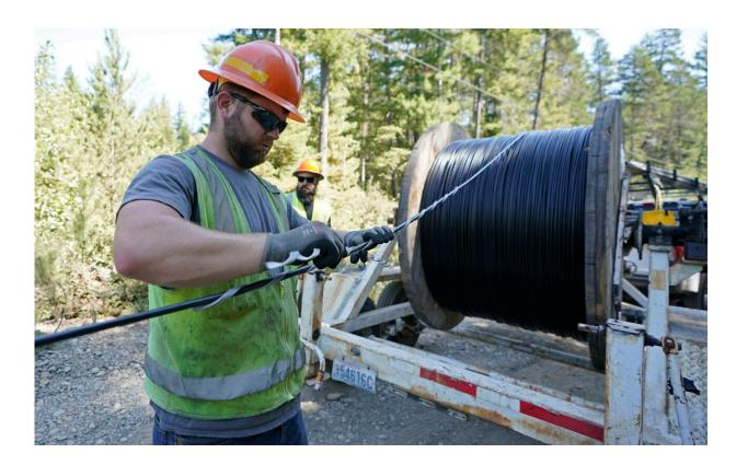
In this Wednesday, Aug. 4, 2021, file photo, Skylar Core, right, a worker with the Mason County (Wash.) Public Utility District, installs a hanger onto fiber optic cable as it comes off of a spool, while working with a team to install broadband internet service to homes in a rural area surrounding Lake Christine near Belfair, Wash. Credit: AP Photo/Ted S. Warren, File
