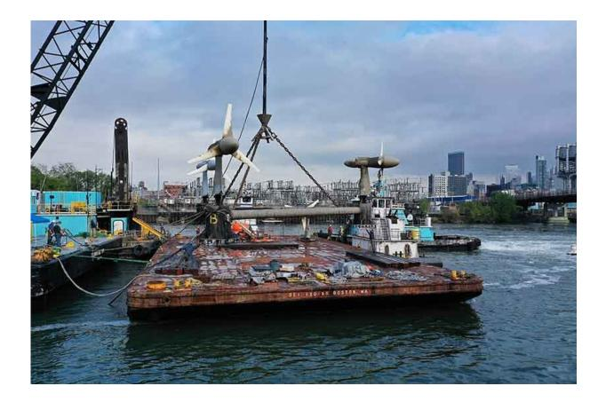
In May 2021, Verdant Power performed a retrieve-and-replace operation, during which one of the turbines will be replaced with a rotor housing three thermoplastic blades manufactured by NREL. Credit: Paul Komosinski
