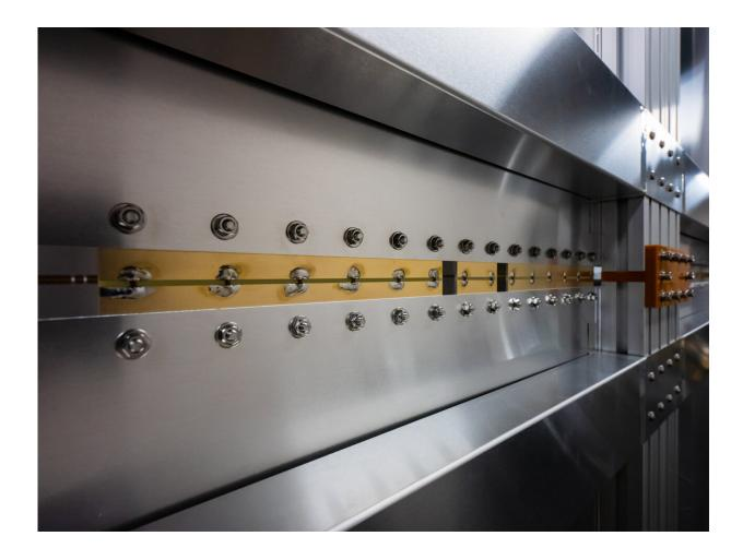
Lumped capacitors set into wall cavities in the wireless charging room. Credit: The University of Tokyo
