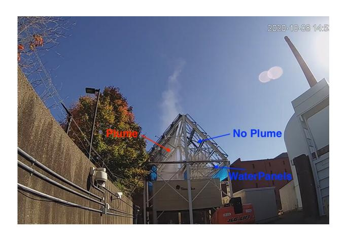
The cooling tower of MIT's nuclear plant has demonstrated the effectiveness of the new water recovery system. The right side of the tower has the new system installed, eliminating its plume of vapor, while the untreated left side continues to produce a steady vapor stream. Credit: Massachusetts Institute of Technology
