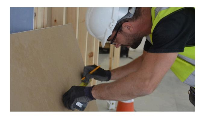
Adaptavate is developing biodegradable plasterboard that is made using crop waste instead of gypsum. Credit: Adaptavate
