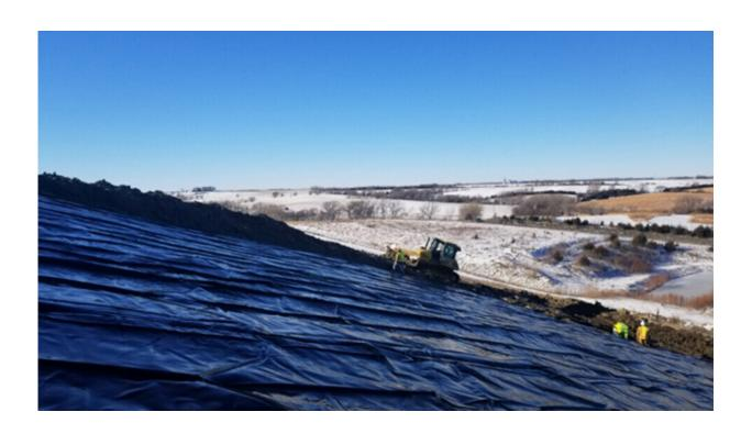
Husker researchers are testing a new landfill ground covering system shown to improve landfill gas emissions. Credit: University of Nebraska-Lincoln
