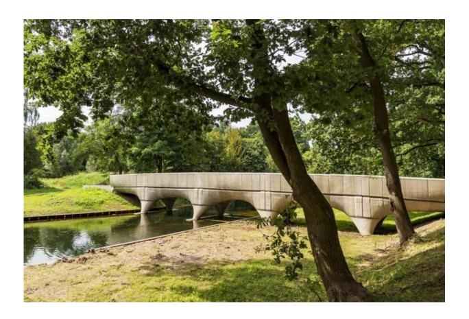
The 3D-printed concrete bicycle bridge in Nijmegen. Credit: Municipality of Nijmegen
