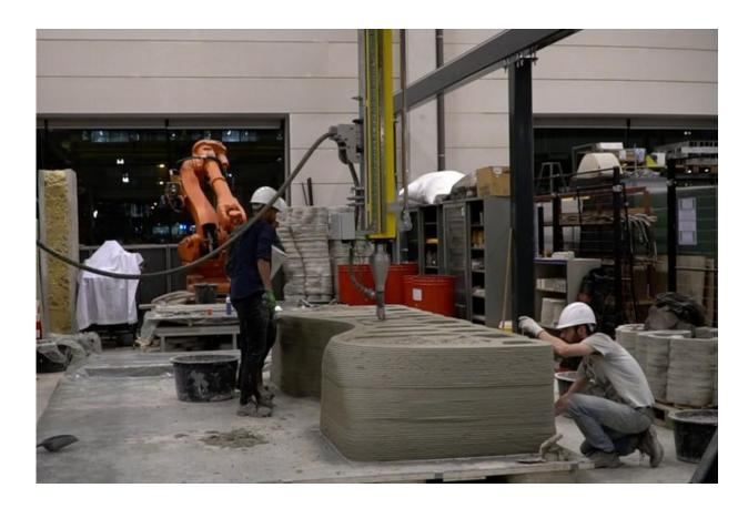
The bridge was printed layer by layer in the concrete printing plant. Credit: Michiel van der Kley
