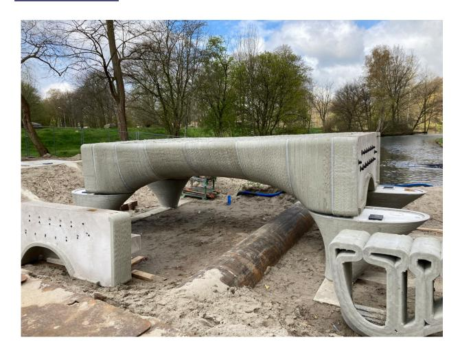
During the printing process, the choice was made to divide the bridge into printable parts. Credit: Michiel van der Kley
