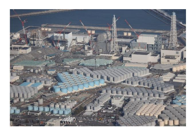
An extensive pumping and filtration system removes most radioactive elements from the water stored at the Fukushima plant.
