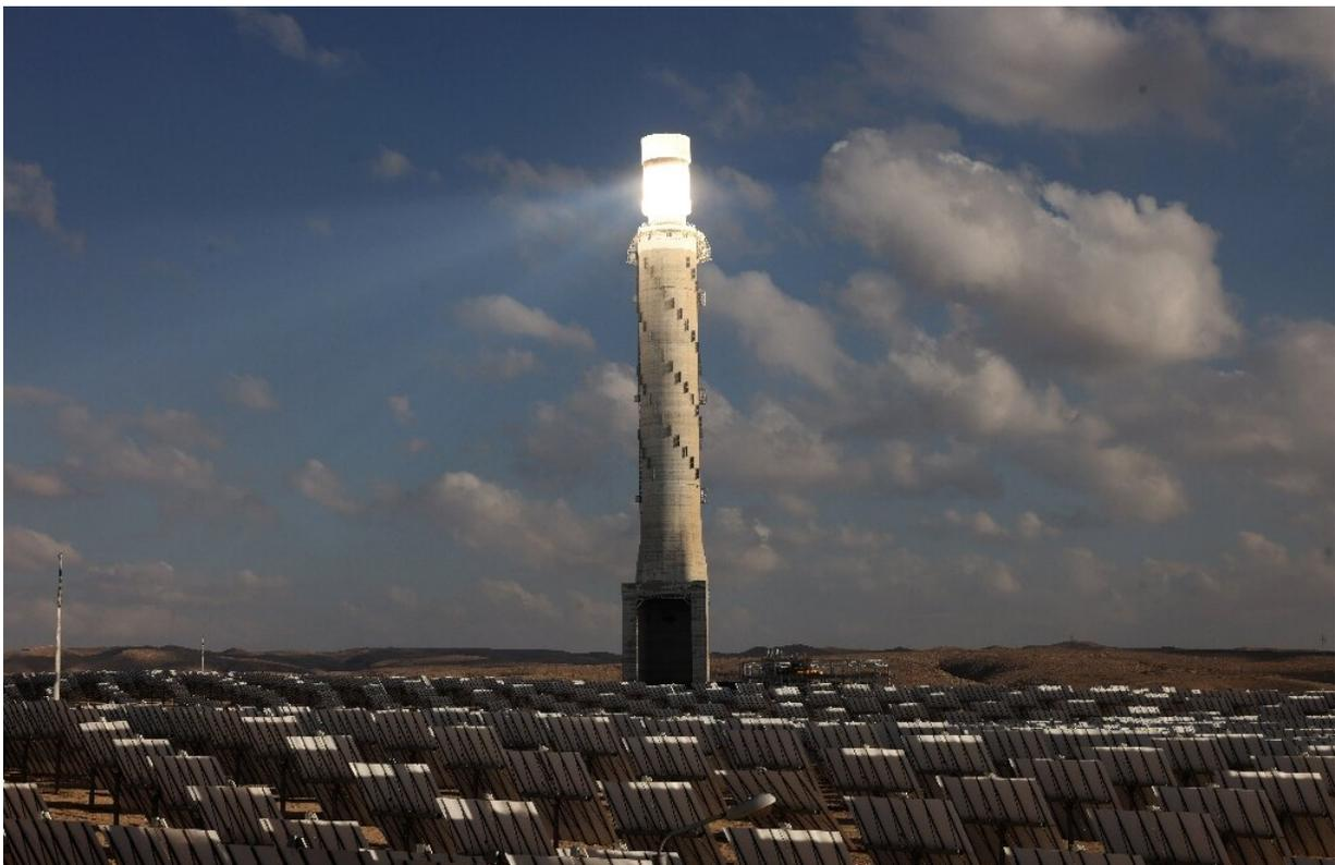
The solar tower of Israel's Ashalim power station, is surrounded by solar panels, in the Negev desert near the kibbutz of the same name, on September 27, 2021. The 240-meter tower is part of a 121-megawatt solar thermal power plant which concentrates the sun's heat from thousands of small mirrors onto a boiler mounted on the tower, the latter producing high-temperature steam used to generate electricity.
