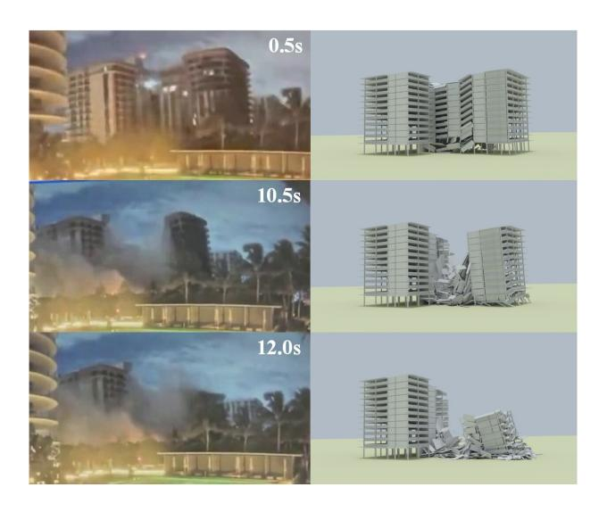
Comparison between actual and simulated collapse process. Credit: Andy Slater
