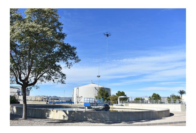
An electronic nose on a drone collects air for odor measurement. Credit: Maria Deseada Esclapez
