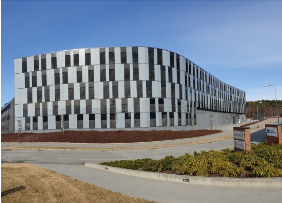
BIPV at the Norwegian Petroleum Directorate. Credit: Hassan Gholami
