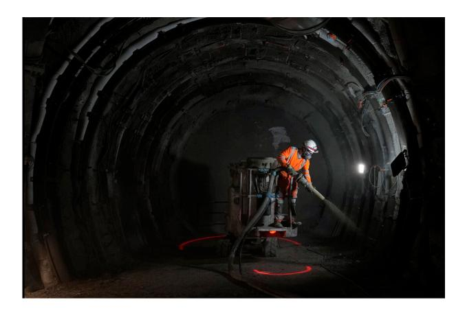
A worker sprays a layer of cement protection in a tunnel for radioactive waste in an underground laboratory run by Andra, an agency that manages the waste, in Bure, eastern France, Thursday, Oct. 28, 2021. Nuclear power is a central sticking point as negotiators plot out the world's future energy strategy at the climate talks in Glasgow, Scotland. Credit: AP Photo/Francois Mori
