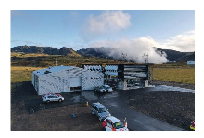
The Icelandic plant enterprise sucks carbon dioxide from the air using technology that mimics, in accelerated format, a natural process that can take hundreds of thousands of years.
