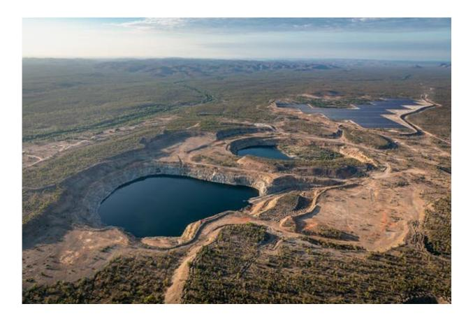
The Kidston pumped hydro project in Australia uses an old gold mine for reservoirs. Credit: Genex Power
