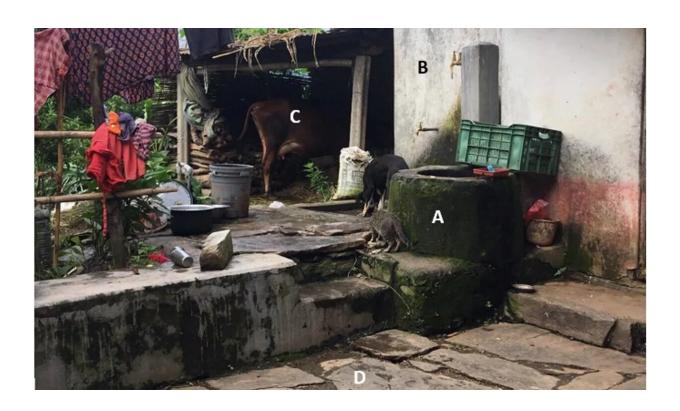
TLAD in Nepali village: cow dung and food waste inlet (A); toilet (B), animal holding and digester (C); digester dome is underground (D). Credit: University of Stirling
