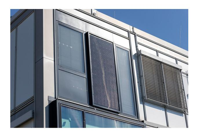
Exterior view of the RE modular facade with a floor-to-ceiling PV element. Credit: Fraunhofer-Gesellschaft
