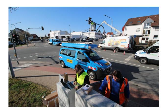
The "KI4LSA" project aims to provide smart, predictive traffic light changing using artificial intelligence. Highresolution cameras and radar sensors gather detailed traffic information. Credit: Fraunhofer-Gesellschaft
