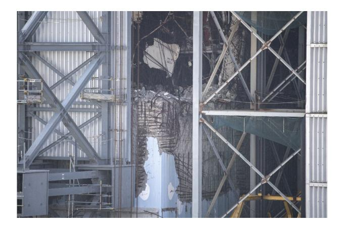
Evidence of the blasts' power is still visible at the top of unit 1, where the warped metal framework remains exposed to the air, and on unit 3 damaged walls stripped of paint sit under a new roof cover.
