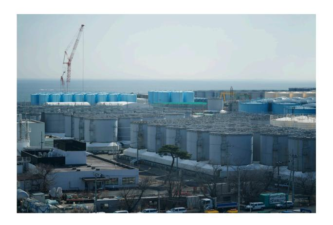
Tanks storing treated radioactive water after it was used to cool the melted fuel are seen at the Fukushima Daiichi nuclear power plant, run by Tokyo Electric Power Company Holdings (TEPCO), in Okuma town, northeastern Japan, Thursday, March 3, 2022. The government has announced plans to release the water after treatment and dilution to well below the legally releasable levels through a planned undersea tunnel at a site about 1 kilometer offshore. Credit: AP Photo/Hiro Komae
