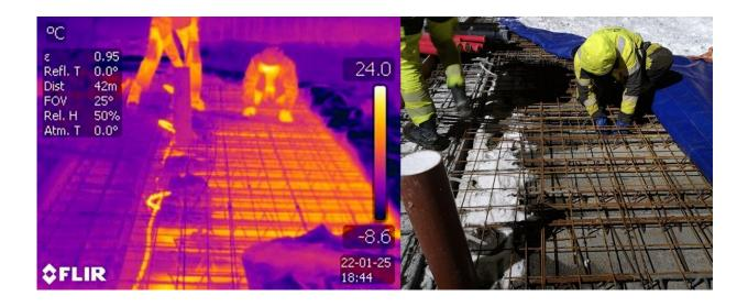
After a few hours of preheating, the cover is pulled aside to make some final adjustments to the reinforcement. The effect of the supplied heat is obvious. Credit: Megan O'Sadnick
