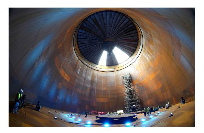
Journalist are seen inside a vast thermal tank to store hot water in Berlin, Germany, Thursday, June 30, 2022. Power provider Vattenfall unveiled a new facility in Berlin on Thursday that turns solar and wind energy into heat, which can be stored in a vast thermal tank and released into the German capital's grid as needed, smoothing out the fluctuating supply problem of renewables. Credit: AP Photo/Michael Sohn
