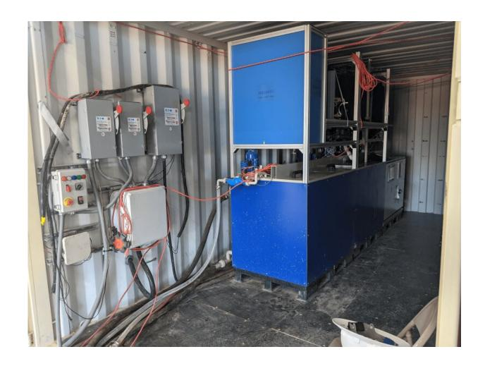
A close-up view of the pilot-scale membrane distillation system. Credit: University of Pittsburgh
