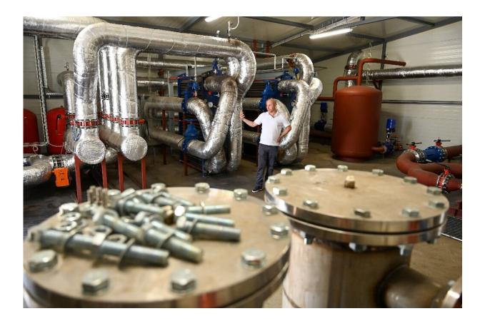
Underground water near the boiling point brought to the surface to heat water running though municipal heating pipes to buildings.
