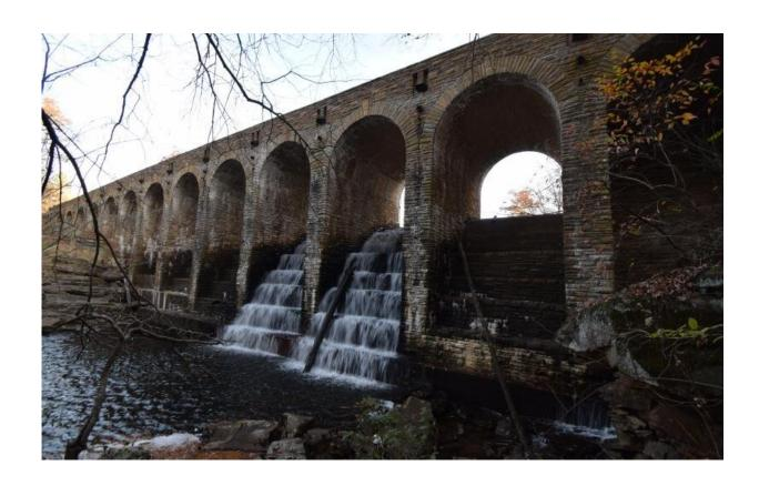
Non-powered dams such as the Byrd Creek Dam in Crossville, Tennessee, may prove viable as retrofitted hydropower facilities, producing sustainable, clean electricity. Credit: Scott DeNeale/ORNL, U.S. Dept. of Energy
