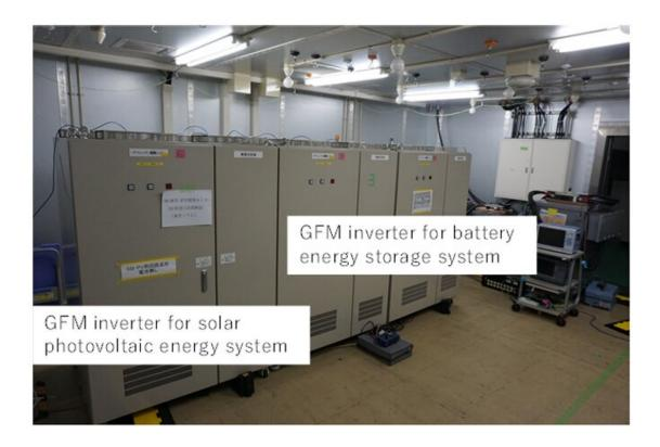
Figure 2: The developed prototype GFM inverter. Credit: Toshiba Corporation News Releases
