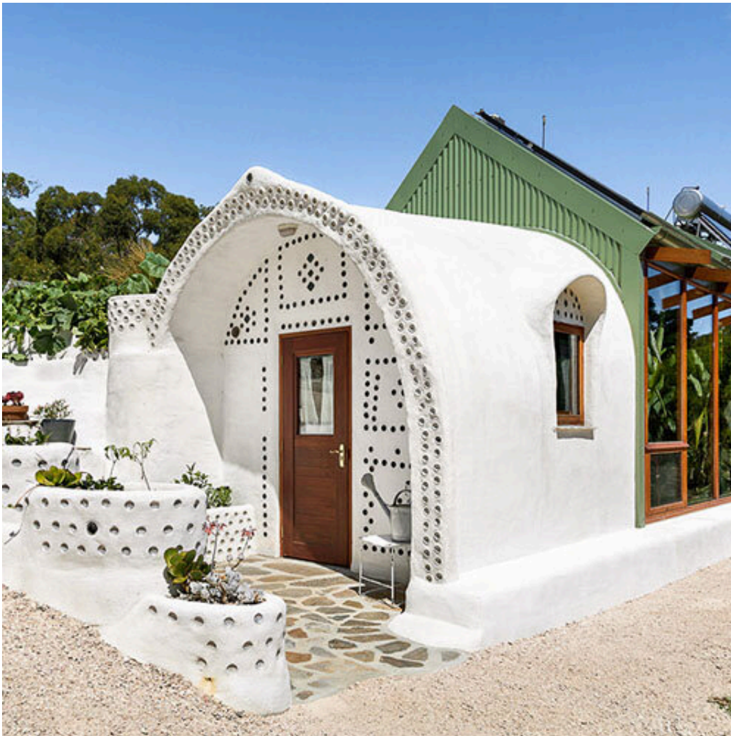
"Earthship" built from recycled tires at Ironbank, SA.
